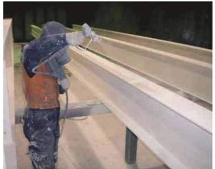
Application on solid I-beam
